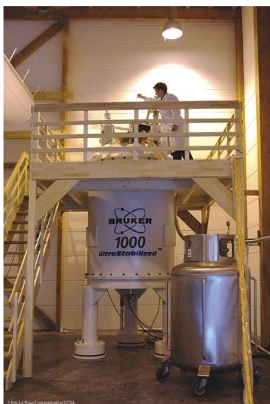
installation in Lyon
