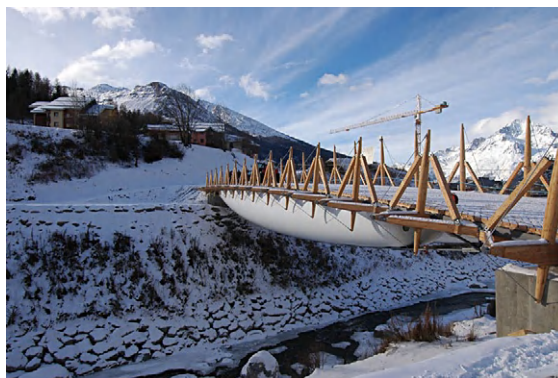
FIGURE 13.10 The Lanselevillard bridge in the Alps spanning 52 m. A very low-weight structure is achieved using the tensairity principle where airbeams stabilize compression and tension elements. Such a structure would benefit from a self-sealing mechanism using a principle inspired by the twining liana Aristolochia macrophylla . Currently, the self-sealing mechanism has only been tested on demonstrator constructions. Photograph reproduced with kind permission from Dr. Rolf Luchsinger, Empa—Center for Synergetic Structures.
